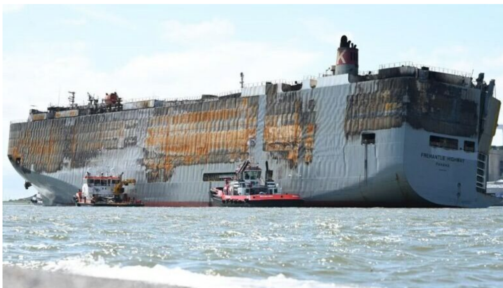
Pic.2 Fremantle highway fire accident
