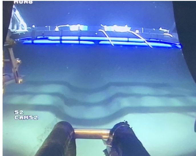
Pic. 2. Cable trench after burial
